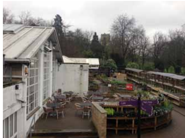
TERRACE LOOKING NORTH TO ALEXANDRA PALACE
